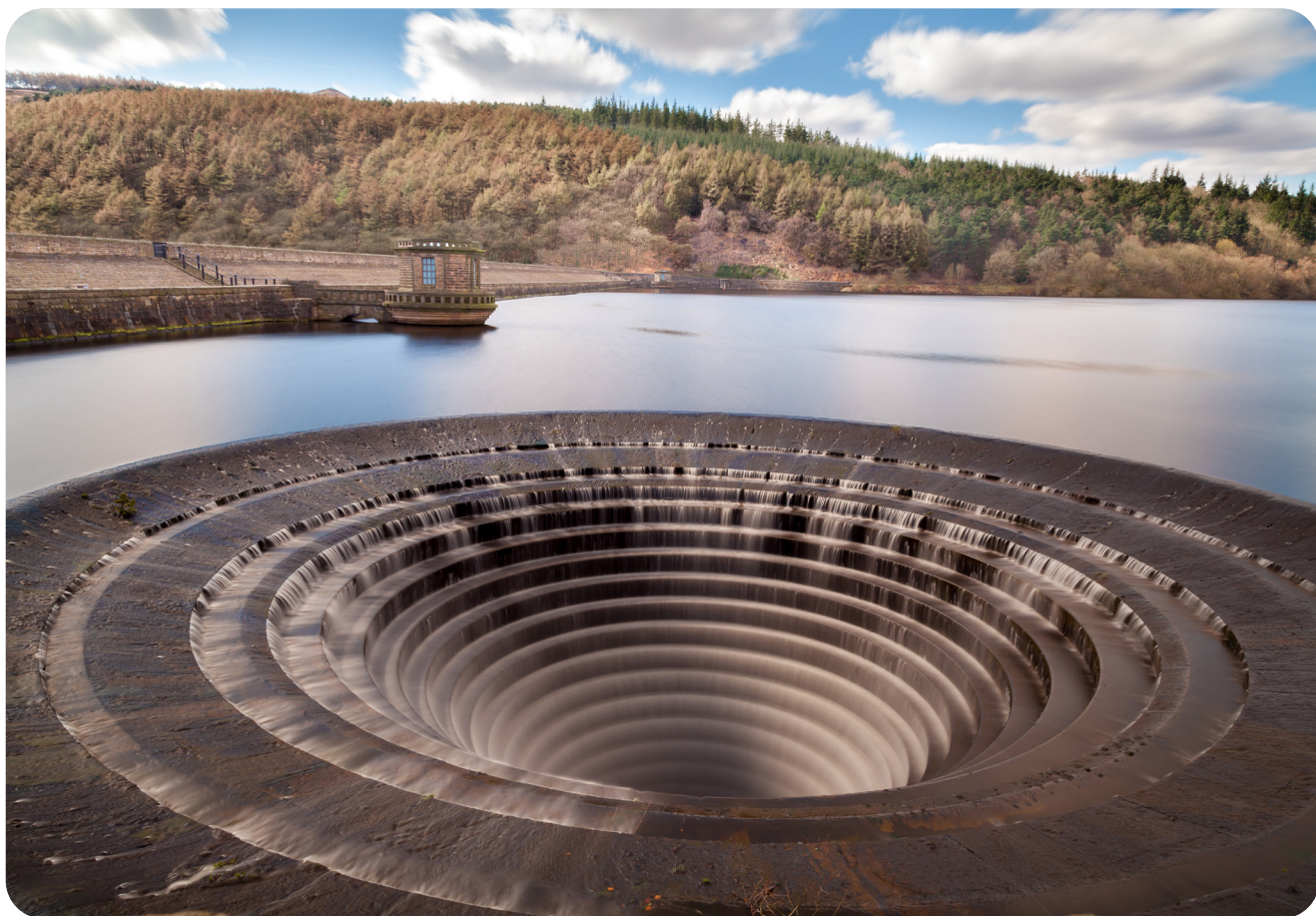
The overflow 'plughole' at Ladybower Reservoir in Derbyshire, England
