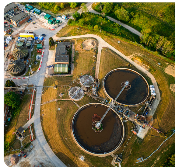
Upgrading water infrastructure – such as this sewage treatment facility in southeast England – and building long-term resilience will require substantial investment
