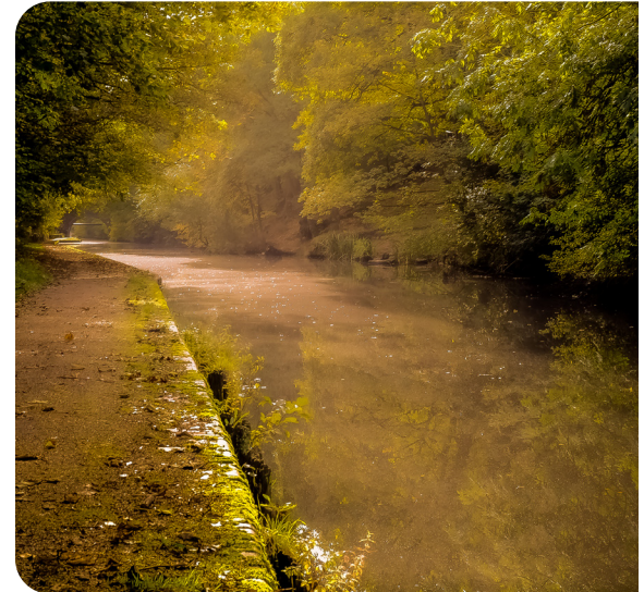
The Grand Union Canal scheme, delivered by Affinity Water and Severn Trent Water, links new pipelines with canal infrastructure to transport water across regions as part of a wider supply and resilience programme
