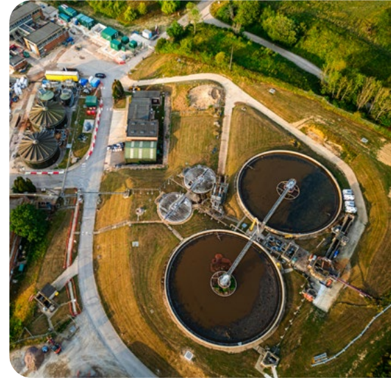
Upgrading water infrastructure – such as this sewage treatment facility in southeast England – and building long-term resilience will require substantial investment
