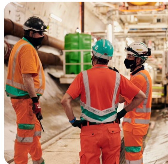
Under construction between 2015 – 2025, the Thames Tideway Tunnel was a trailblazing example of how to deliver water infrastructure differently
