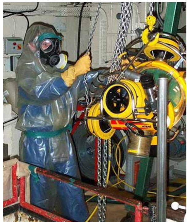
Using remotely operated vehicles to help in the cleaning up of legacy ponds and silos
