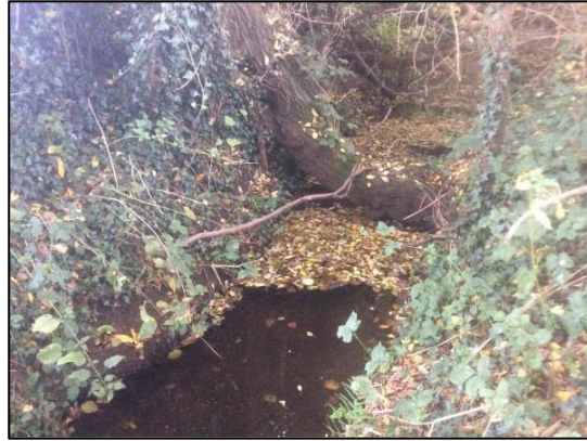
Downstream view taken from SK 08096 19253
