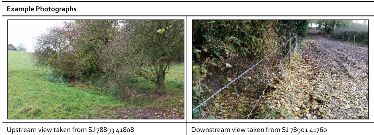
Figure 49: Example photographs taken during field survey of Unnamed tributary of River Lea 2
