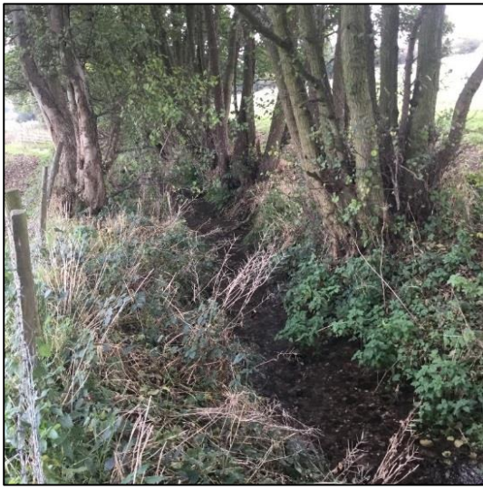
Upstream view taken from SK 05171 21307
