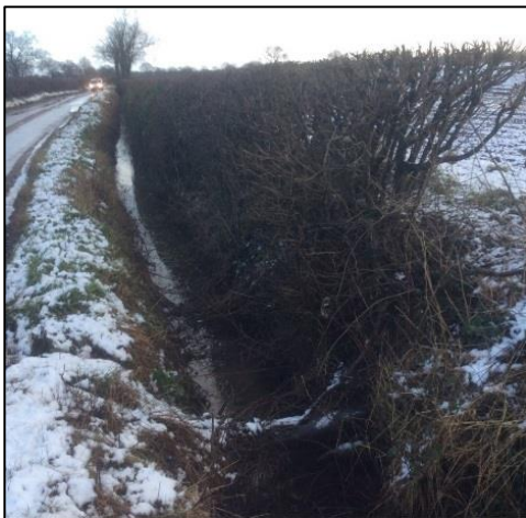
Downstream view taken from SK 09859 17887
